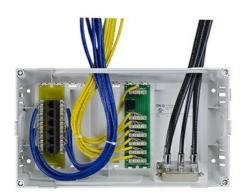
This patch panel provides a termination point for up to six Ethernet drops. It is designed to be specified into an EN0800 enclosure for basic structured wiring applications, such as multi-dwelling units and small homes.
